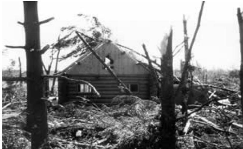
At door and window openings, the logs had been twisted clockwise (viewed from the top), and the openings the logs stepped out 1/8" to 1/4" per round. Every layer of logs moved, right down to the bottom sill logs. Door openings had about 2" out of plumb from top to bottom.
