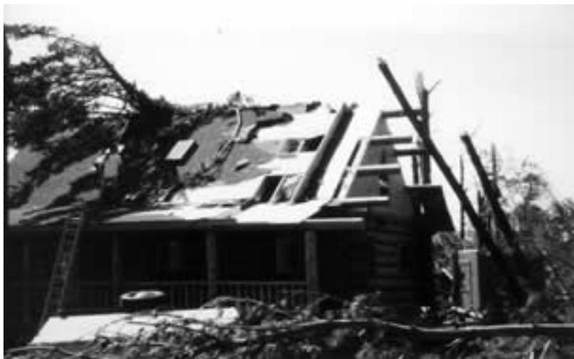
2x12 common rafters to the purlins with 4" and 6" pole barn (ring shank) nails. At the ridge, the common rafters were overlapped and spiked to each other and to the ridge log. OSB sheathing was used as the roof deck for shingles.
